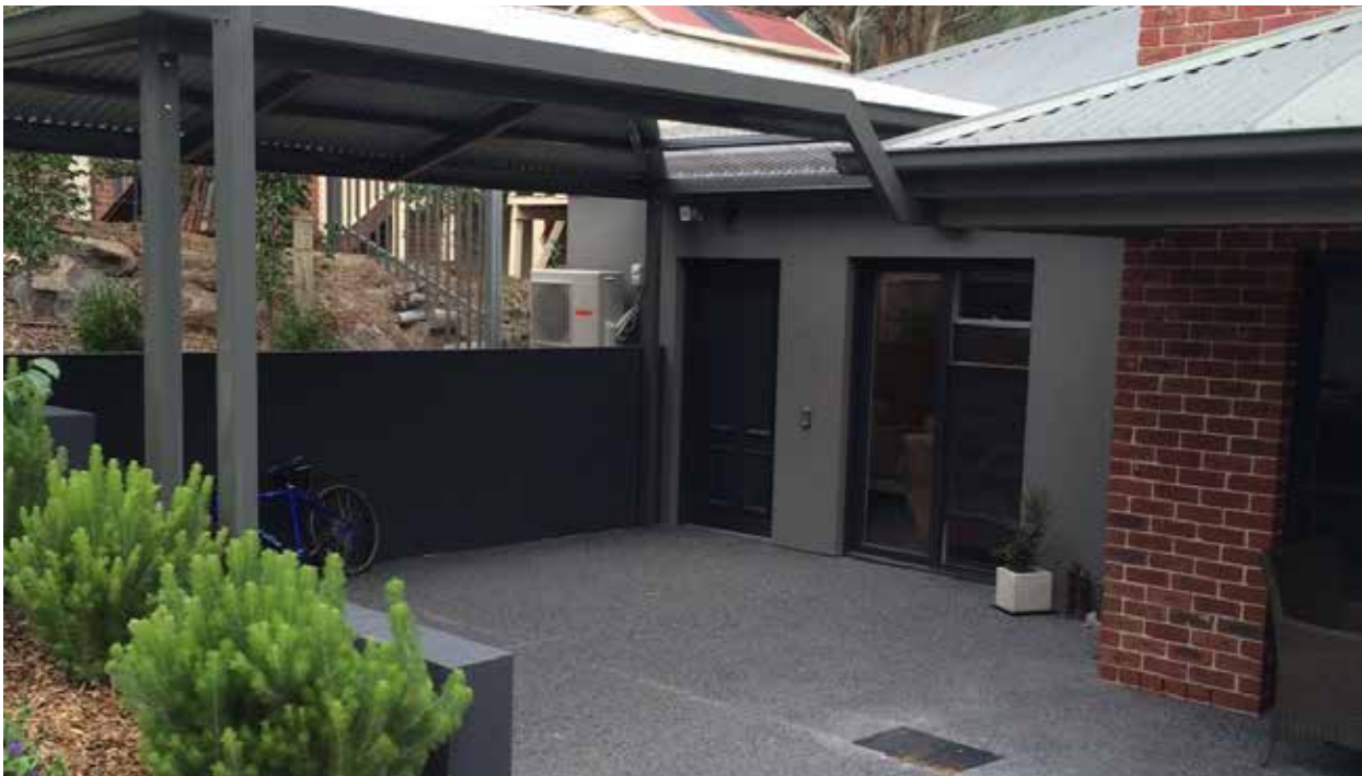
Covered accessible car space with generous overhead clearance and direct covered link to the dwelling, private residence.
