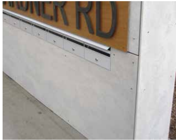
Letterboxes located at an accessible height, Mission Australia (Victoria) housing, MSM Architects.
