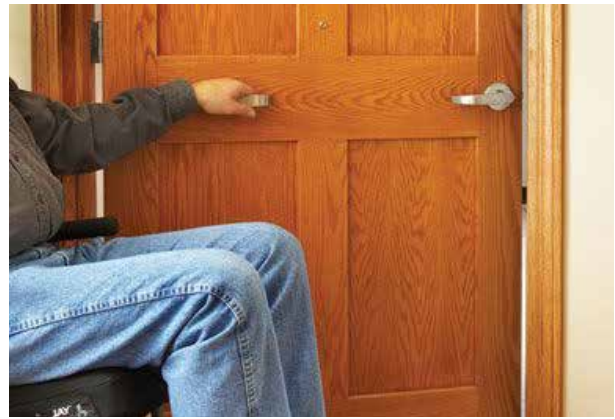
Above: A horizontal handle or pull-bar on the closing face of an outward swinging door can support a person using a wheelchair in closing the door behind them. Such additional controls can be easily added to internal hinged doors as customisations for individuals, if needed.
