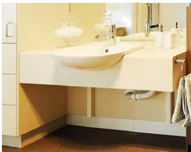
Height adjustable basin and vanity, Hunter Housing Project.
