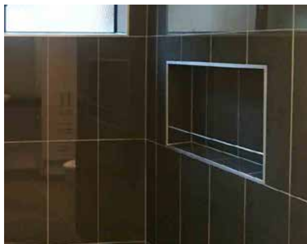
LEFT: Recessed shower shelf located in a corner, for convenient access from a fold-down seat. RIGHT: Recessed shower shelf with steel rod, to prevent items falling on the floor.
