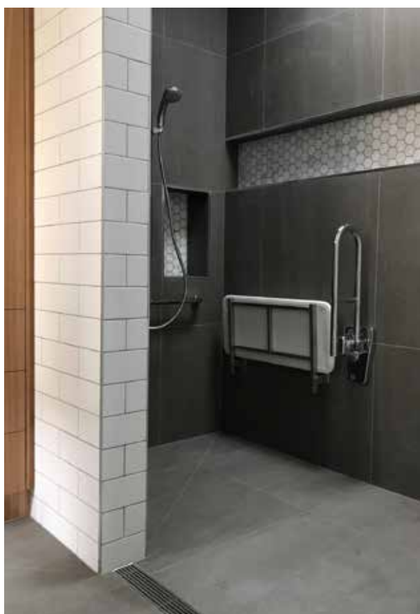
LEFT: Recessed shower shelf located in a corner, for convenient access from a fold-down seat. RIGHT: Recessed shower shelf with steel rod, to prevent items falling on the floor.
