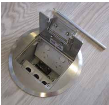
LEFT: In-floor GPO to possible island bench locations, Hunter Housing Project.
